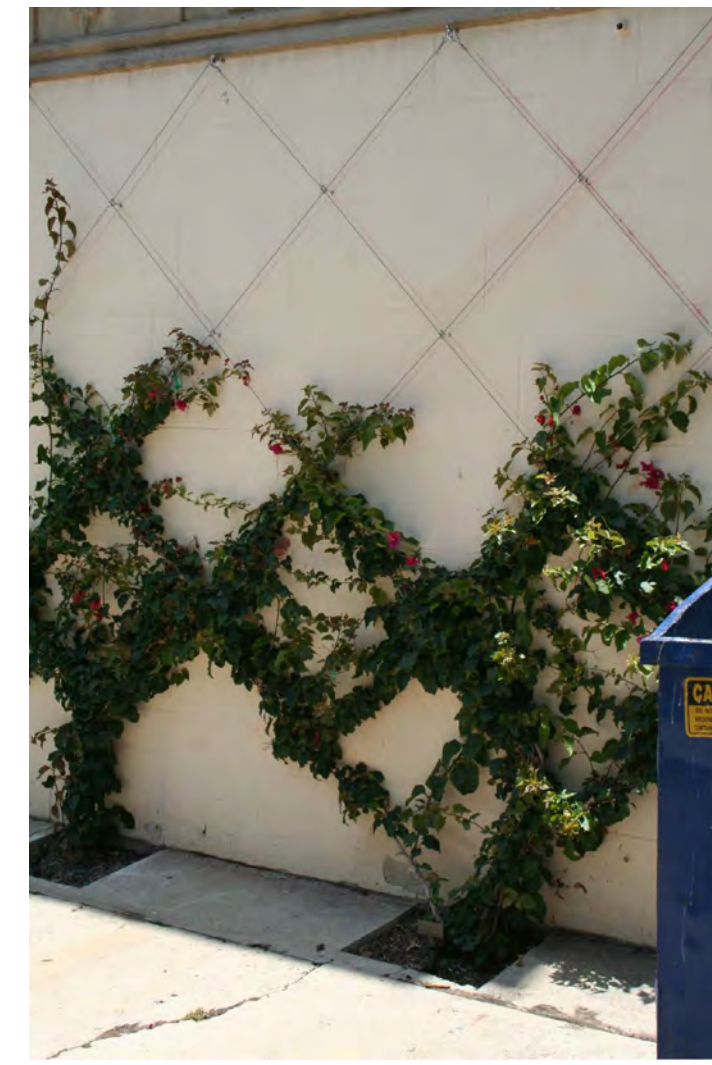
VINE CABLE TRELLIS SYSTEM DIAMOND PATTERN
